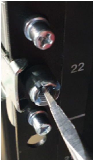
Figure 29. Securing the front of the rails
