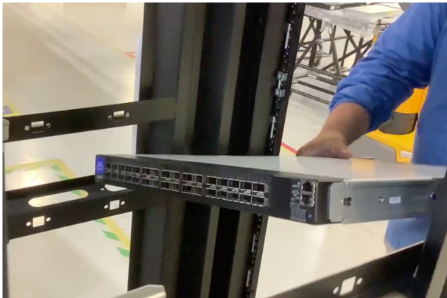
Figure 105. Tilting the switch enclosure to install it
