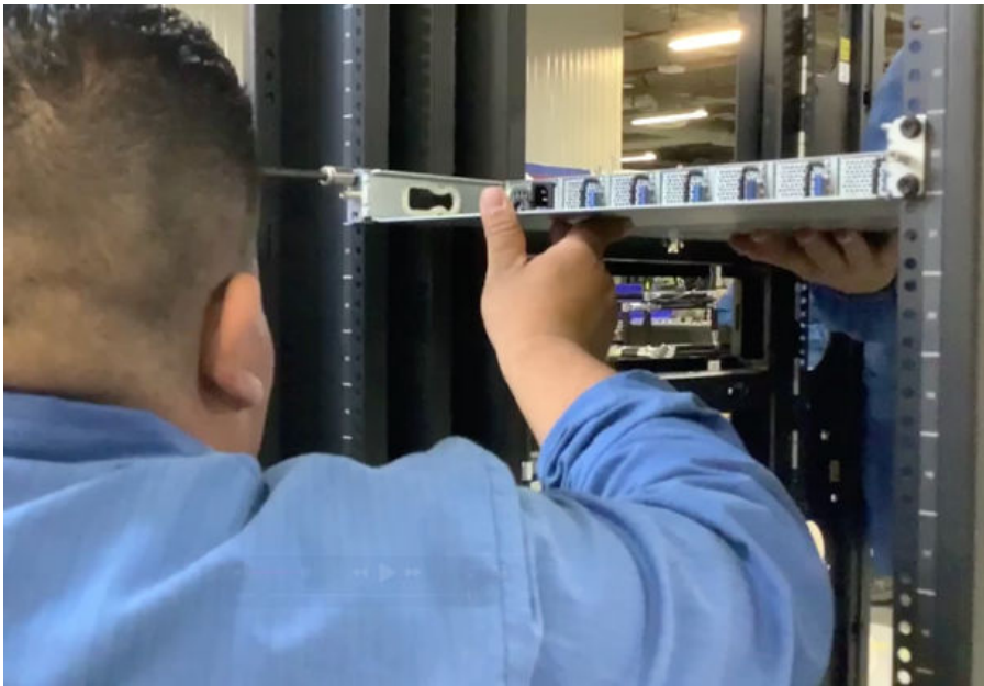
Figure 107. Securing the rack mounting rail
