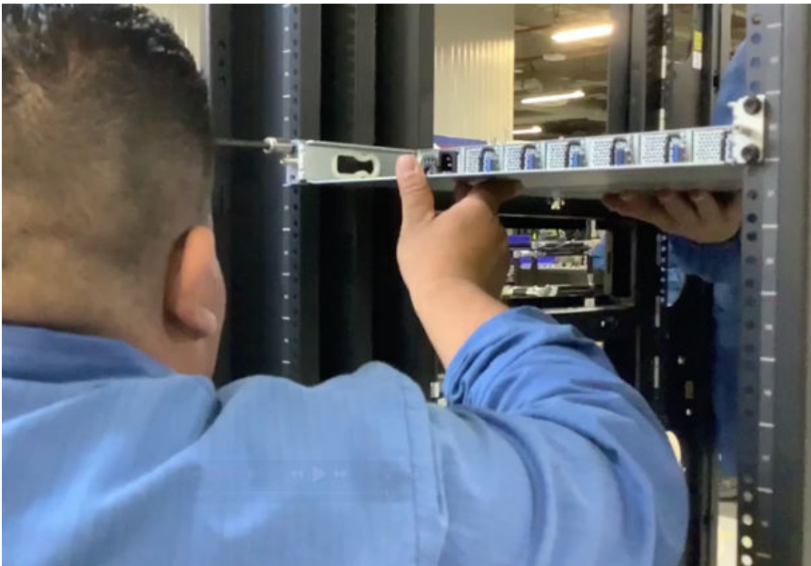
Figure 113. Removing the securing hardware
